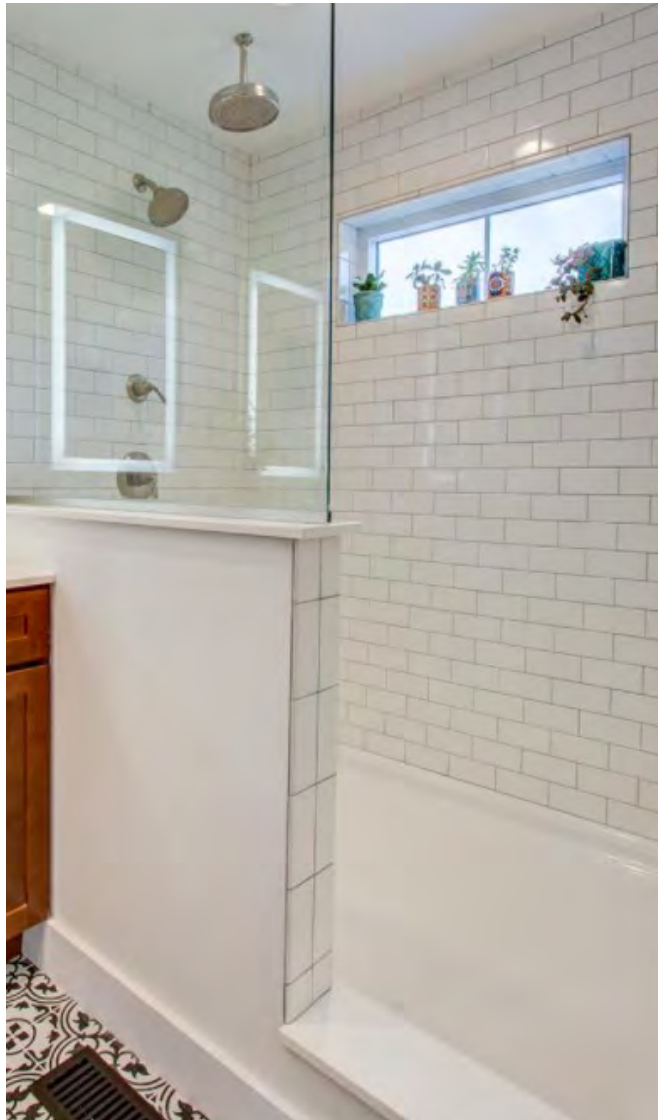
Artic White Tile with Upgraded Faucets
